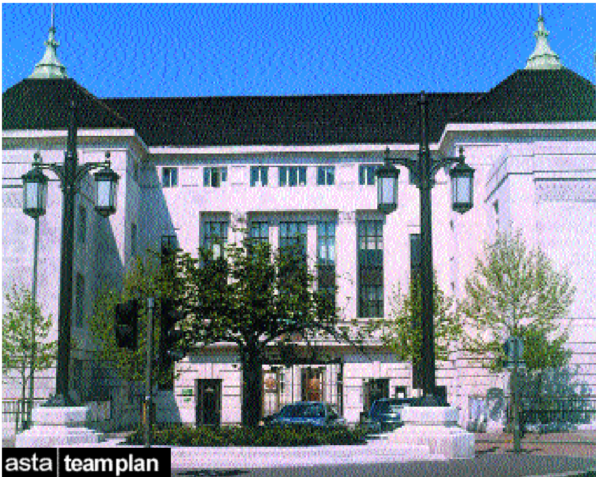
Wandsworth Town Hall, London
